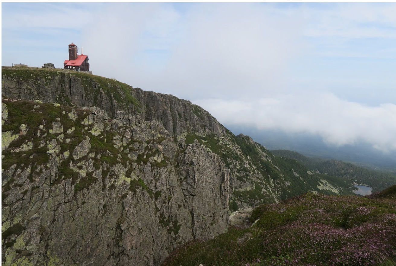
Telecoms station at Snezne
