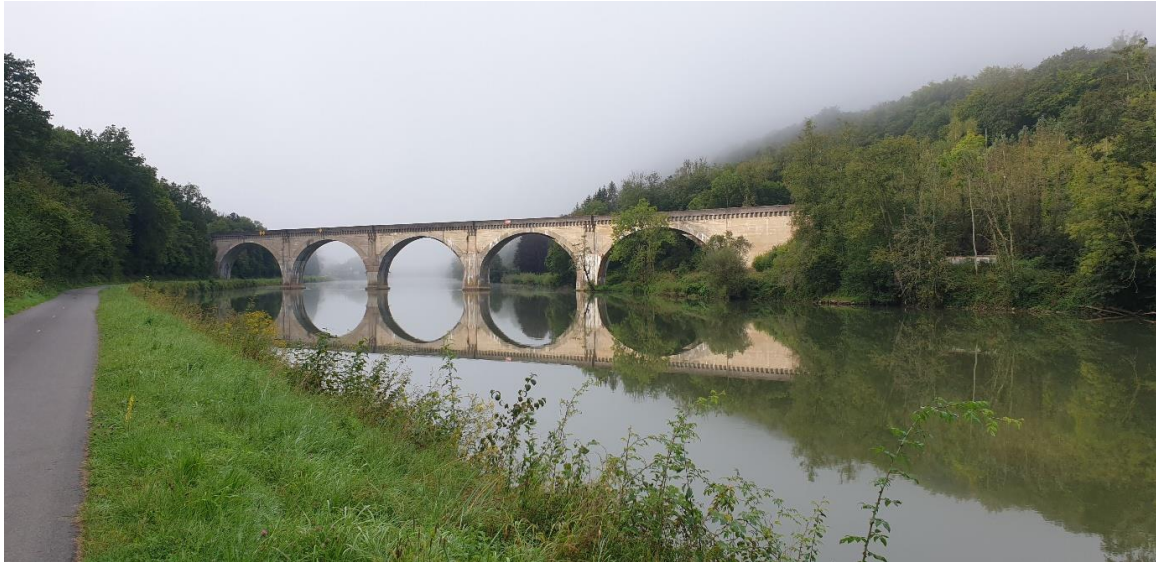
Bridge over the Meuse, France
